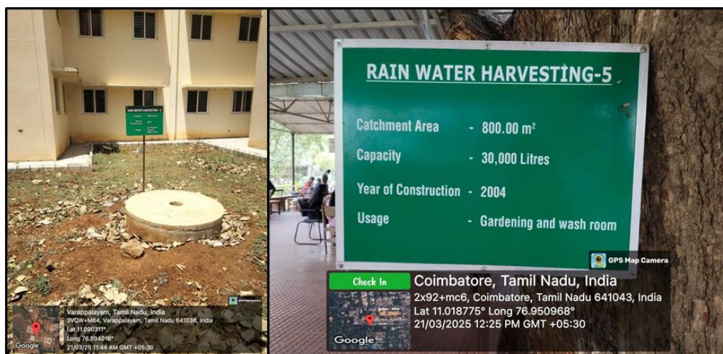
Rainwater harvesting system observed inside the campus
