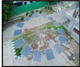
Fig. 4. A view of optimized solar power plant
