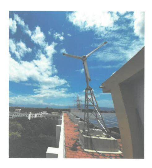
The Wind turbine at the roof of Library Block in the main campus is a source of wind energy which generates 1 KW energy. This is one of the alternate energy source adopted by the institution.
