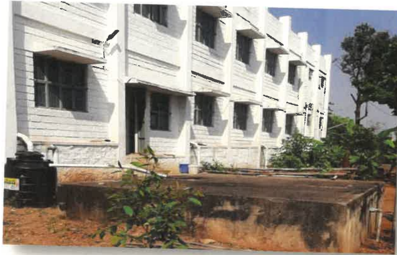
Rain Water collection tank (Campus II)
